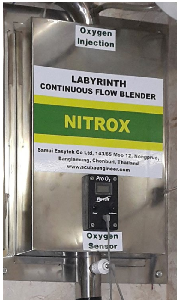
Continuous flow nitrox blender... still in the future
